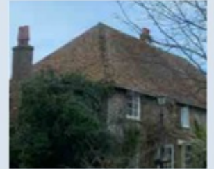
Clay plain tile hipped roof
