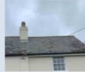
Slate tile pitched roof
