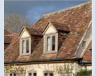
Kent peg tiles in light/red brown and gabled dormers
